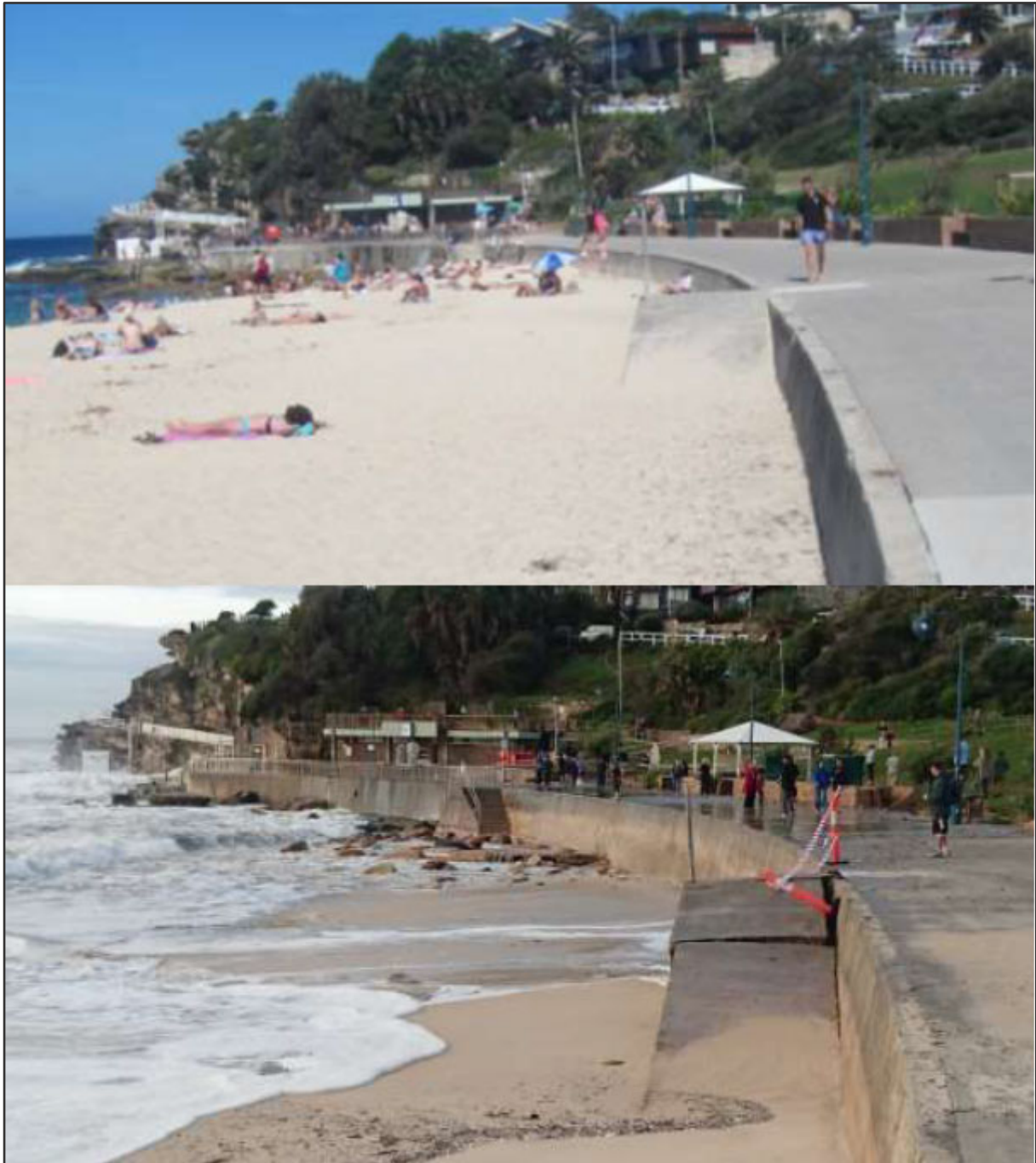
Figure 5-8 View of southern length of Bronte Beach and seawall showing differences in beach profile before (top image, 1 April 2016) and immediately after (bottom image, 6 June 2016) the East Coast Low storm event (source: (ARUP, 2016) (top), (Baird, 2016) (bottom)).
