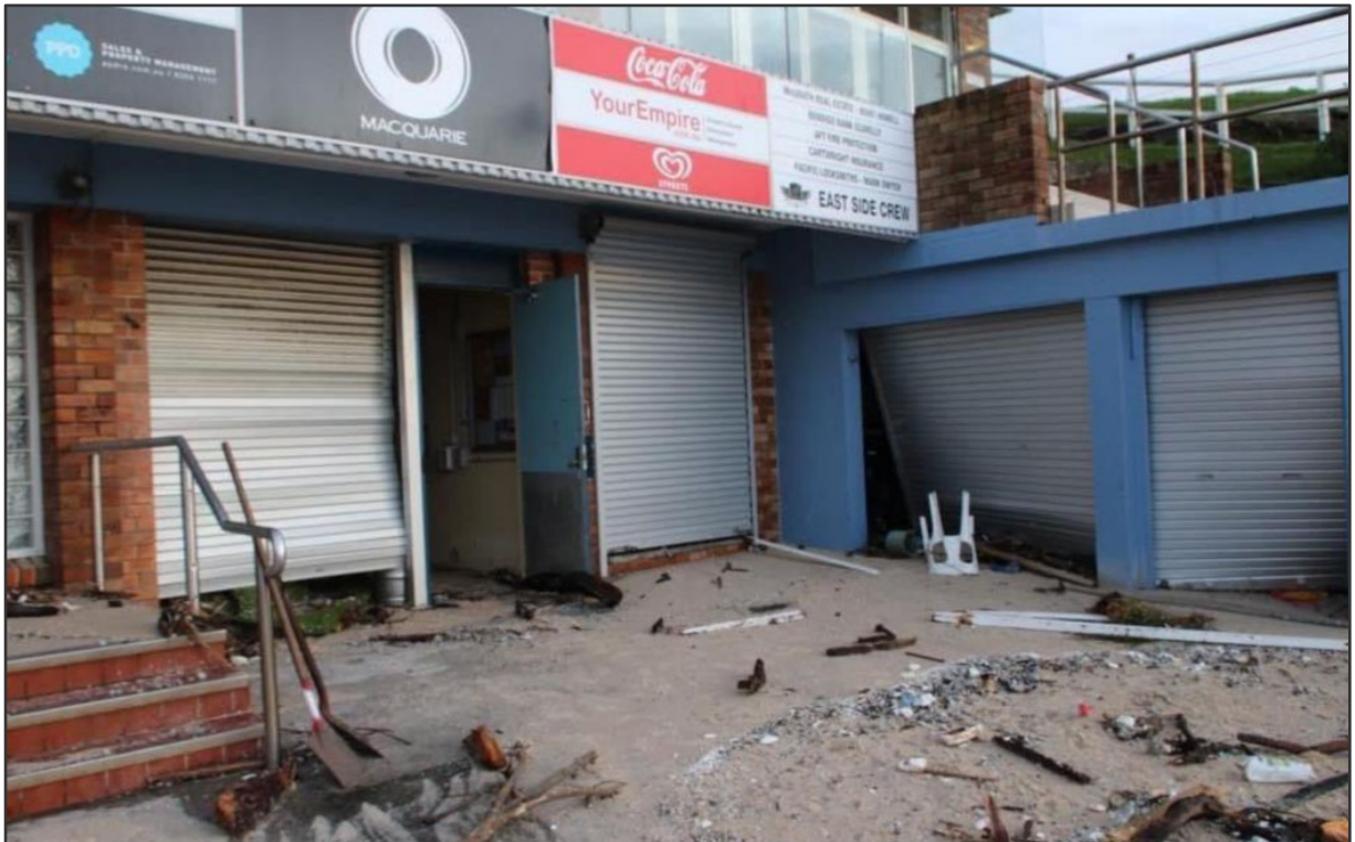
Figure 2-6 Damage to roller doors at Bronte SLSC in June 2016
