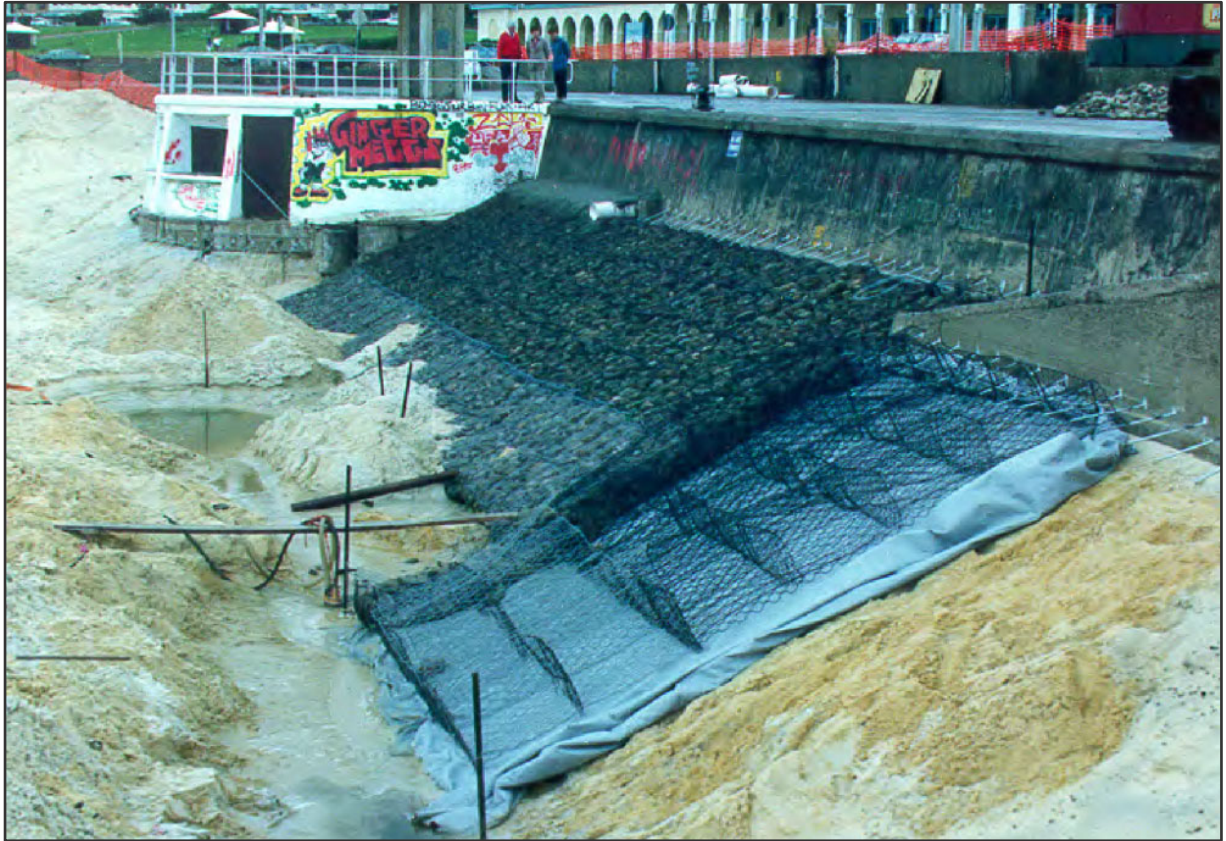
Figure 2-5 Construction of Bondi seawall reno-mattress toe protection 1987 ( (WorleyParsons, 2011))
